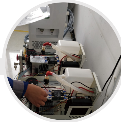
Second inspection Electrical line inspection
